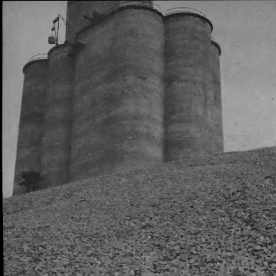
Shelled corn towers alongside the 175-foot high elevator and its 21 bins which can store 350,000 bushels of grain.
