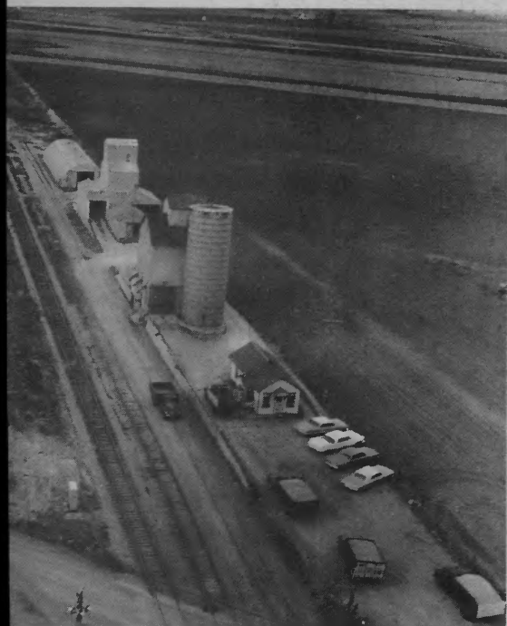
Truckloads of corn pass over the old scales until work is finished on the new $340,000 elevator.
