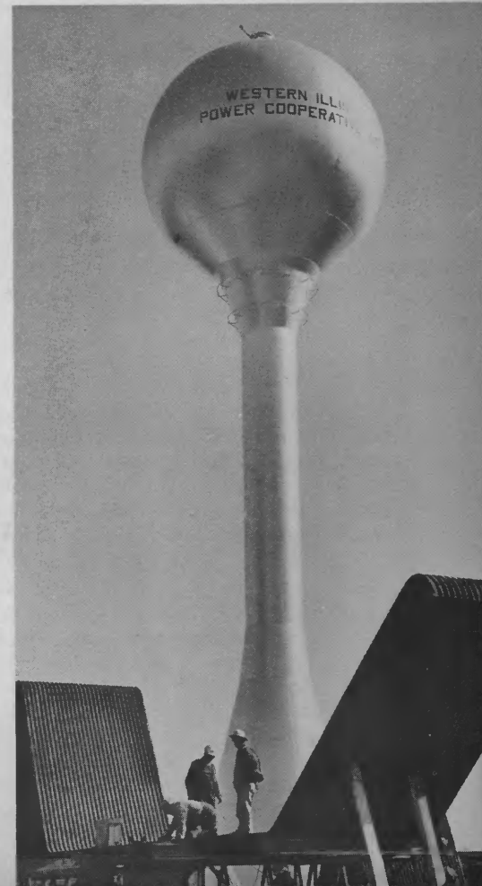
A thing of beauty is this 100,000-gallon WIPCO water storage tank.
