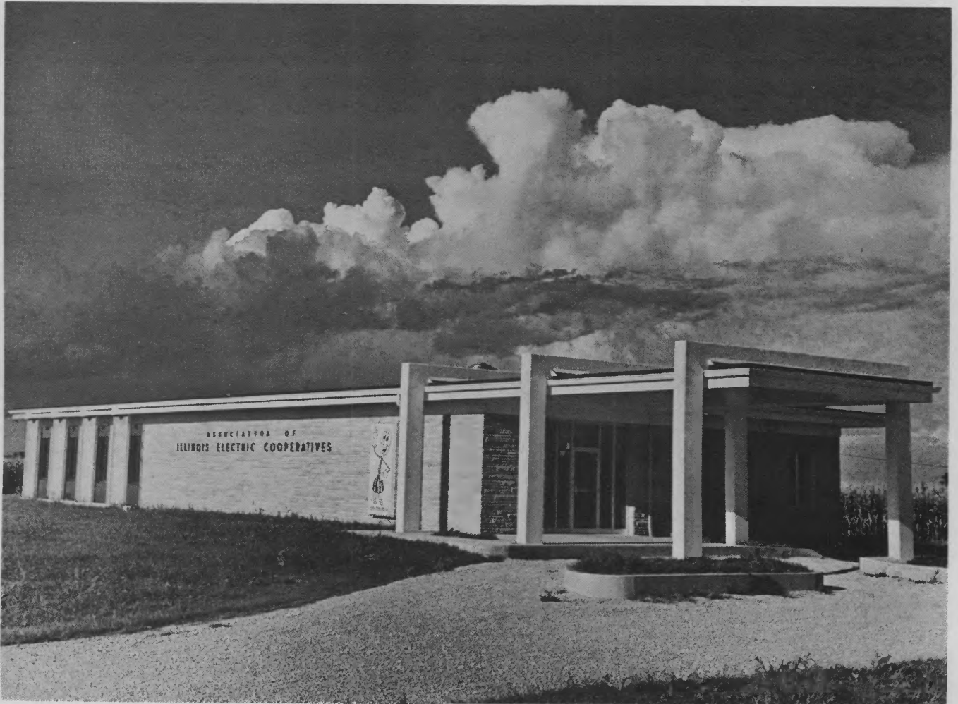
NEW HEADQUARTERS OF ASSOCIATION OF ILLINOIS ELECTRIC COOPERATIVES
