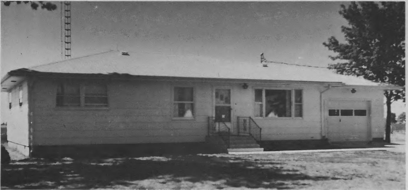
The new "all-electric" Gold Medallion home of Mr. and Mrs. Archie Hawkins located southeast of Taylorville.
