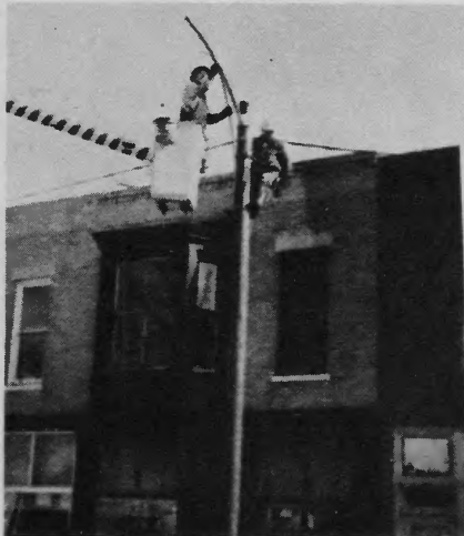
Earl Westenhaver and Delmar Brunk installing one of 68 mercury vapor lights in the Village of Cowden.
