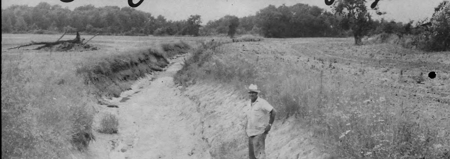
JOHN D. BAYLOR RECLAIMED SOME BOTTOM LAND BY WIDENING AND STRAIGHTENING OUT A CREEK BED.
