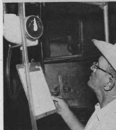
Robert turns a control and the entire washing operation of milkers and pipeline is handled automatically without any more attention.
