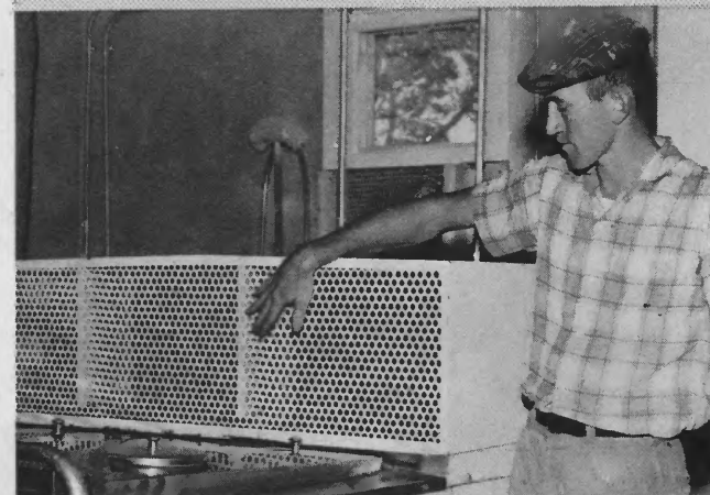
The Hollaways expect to warm the milk room of the new dairy building in winter with heat generated from the compressor of the bulk tank.
