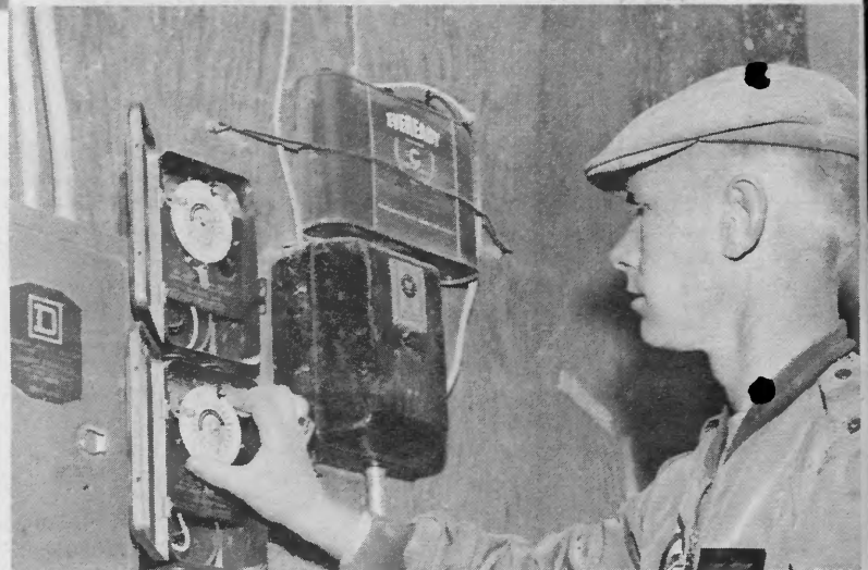
Time switches control four rows of 80 fluorescent lamps, each set to go on at five-minute intervals thus conditioning birds to light.
