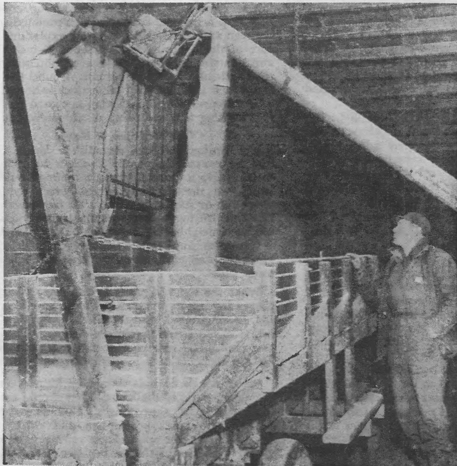
From storage bin to self-unloading wagon, Parks' grain is electrically augered. Hand labor has been eliminated.
