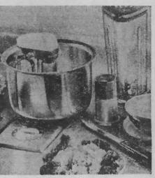
Latest in kitchen equipment is this combination mixer, blender, juicer, and knife sharpener built into the counter top. There are six speeds from the one-fifth horsepower motor, installed below the counter top. When not in use a cover is placed over the drive shaft. The unit occupies an area of only 10 by five inches. It is listed at \$74.95 and is made by the Nutone, Inc., Appliance Division, Cincinnati 27, Ohio.
