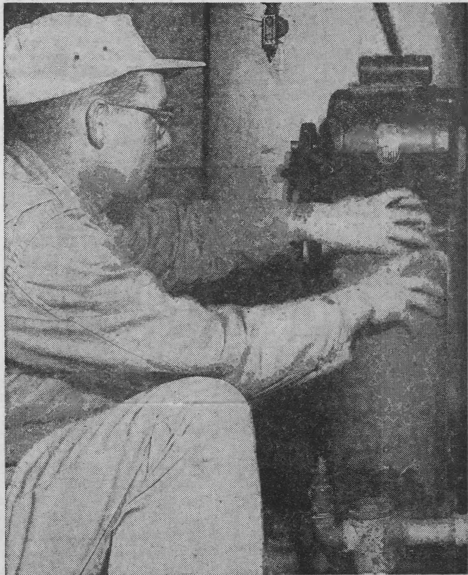
CURTIS BRADLEY laid 1,800 feet of copper pipe from a well to his home because of the availability of electric service. This pump provides the Bradley farm with all its water.
