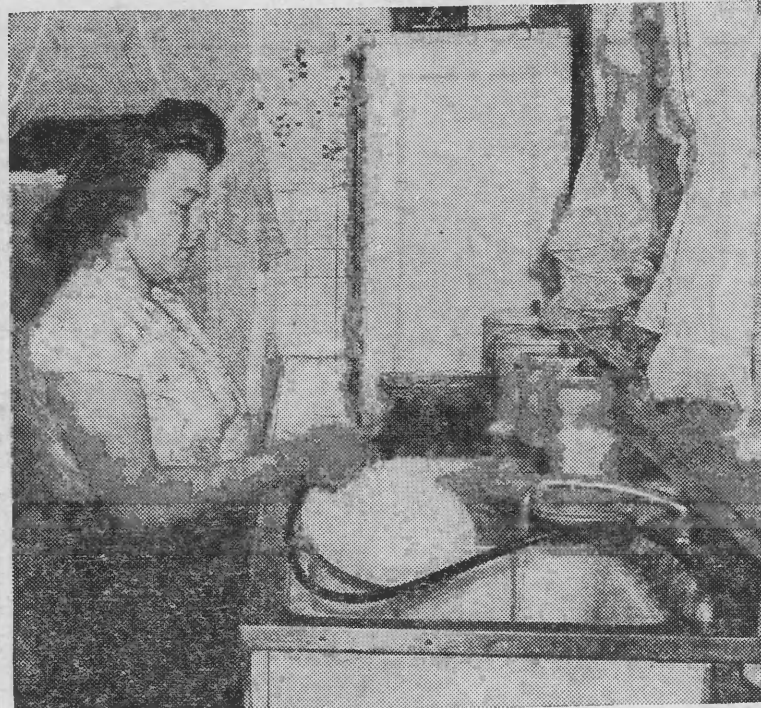
'BIGGEST IMPROVEMENT on our farm' is what the Heckenkemper's of New Baden say about their complete water system. Daughter Myrtle finds dishwashing much easier and pleasanter with hot and cold water at her fingertips. Besides up-to-date kitchen sink, the Heckenkemper's put in a complete bathroom and several hydrants in the out-buildings for the livestock and chickens.
