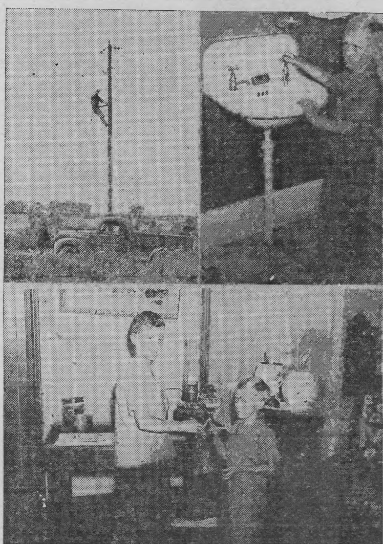
BECAUSE OF THE WORK—pictured in the photo at the UPPER LEFT; water could flow into the wash bowl (UPPER RIGHT), and the job of filling lamps (LOWER PHOTO) passed out of existence. The men at work in the group of pictures are Claude McAfee, on the pole, and William Yost, groundman. The little fellow getting ready to wash his hands (with more pleasure than was ever displayed in a wash basin with water carried in from the pump) is George Dodge, grandson of Mr. and Mrs. Fred Dodge. George, who is seven years old and who spends his summer with his grandparents, is shown BELOW with his playmate, Marion Damm, 13, filling the coal oil lamps for the last time, while workmen prepare to bring service to the farmstead.
