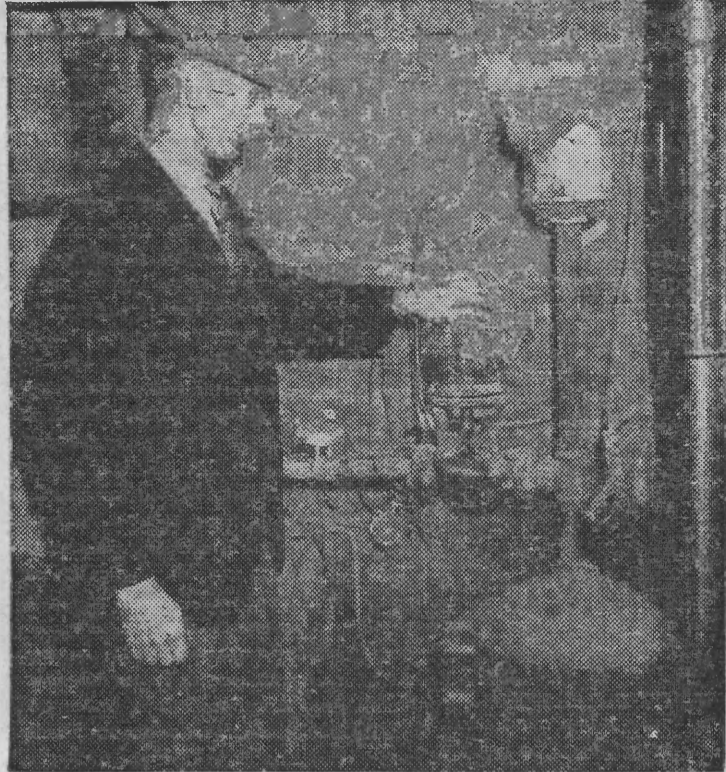
MAKES CHICKENS HAPPY —Mr. Rovie is shown exhibiting the device which keeps his chicken houses at a comfortable temperature throughout the winter. Water, warmed by a coal-burning stove, is circulated by means of a centrifugal pump which Mr. Rovie has his hand on.
