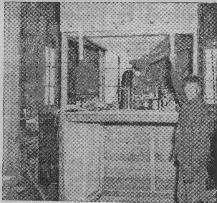
TAKES A HANDY MAN—But, then, that is just exactly what Mr. West is—a handy man if ever there was one. He is shown beside one of his prize home-made pieces of equipment. Shelled corn is dumped into the elevator at the extreme left, and taken to an overhead bin from where it flows by gravity into the hopper (shown at the top, center of the picture), and then down through a feed grinder and into the floor bin. To save scooping the feed out of the floor hopper, Mr. West plans to build an electrically-operated conveyor to take the feed from the floor into an adjoining bin.
