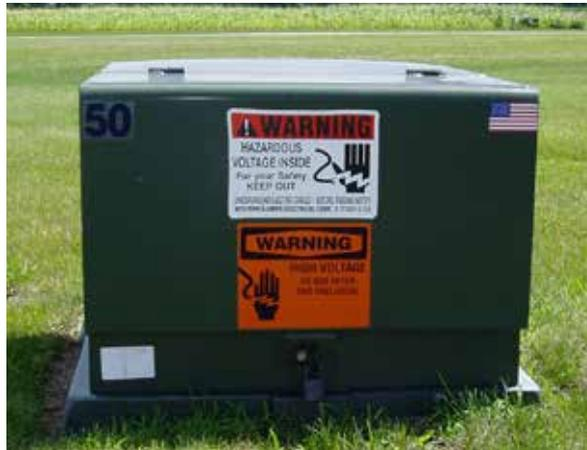
ity flows through this coil, it creates a magnetic field that "induces" a voltage in the other coil. Here is where the magic (aka physics) of transformation takes place. Each coil has a different number of turns. The greater the number of turns, the higher the voltage. The coil on the high side will have
