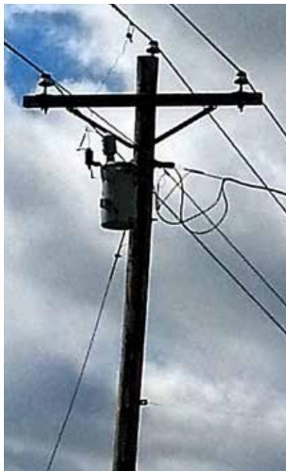
more turns than the one on the low side. As a result, the voltage induced on the low side is less. Then transformation occurs.
