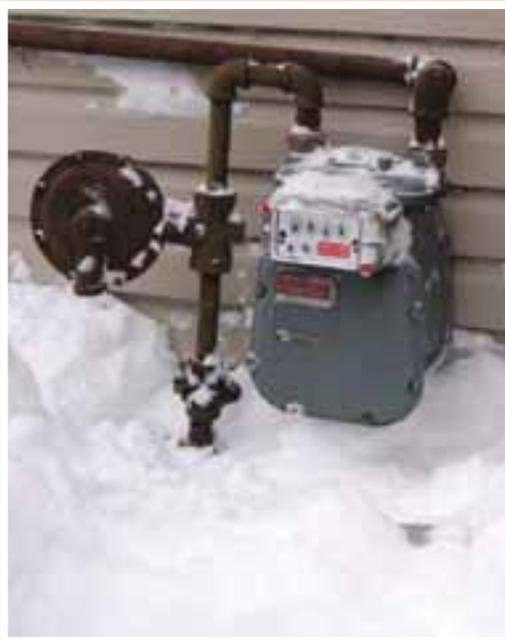
As you're shoveling sidewalks and driveways this winter, remember to check your natural gas meter and pipes for drifted snow, top, which can cause problems. When exposing the meter and pipes, avoid using a snow blower. Instead, gently remove snow and ice from the area.
