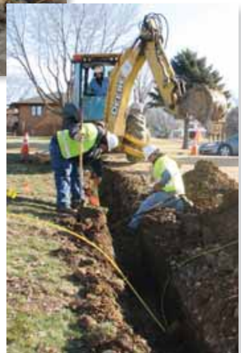
Right: Rock Energy's gas crew installs a natural gas line at a home under construction in Lake Summerset near Davis.
