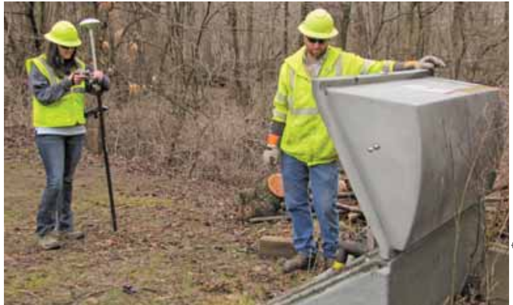
Intern Natalie Pier and lineman Shane Norris check the connections inside an underground enclosure box. They also recorded precise GPS locations for the co-op's equipment to improve the digital mapping system accuracy.
