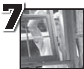
7 New replacement windows
