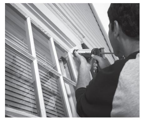
ment means possible air leaks. If you can see daylight around a door or window frame, then the door or window has a leak; you can usually seal these through caulking or weather stripping.
