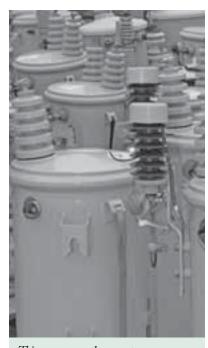
Thieves across the country are damaging electrical equipment like these transformers for the copper they contain. Little do they know that most of the volume of the transformer is insulating oil with very little copper or salvage value. Thieves are risking their lives for a small amount of copper.
