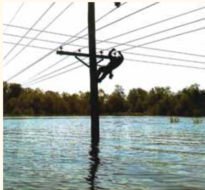
Photo courtesy of Egyptian Electric Cooperative
