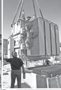
A 98,500-pound transformer was installed at the Sand Ridge substation in August as part of system improvements at the substation adjacent to the Rentech facility.
