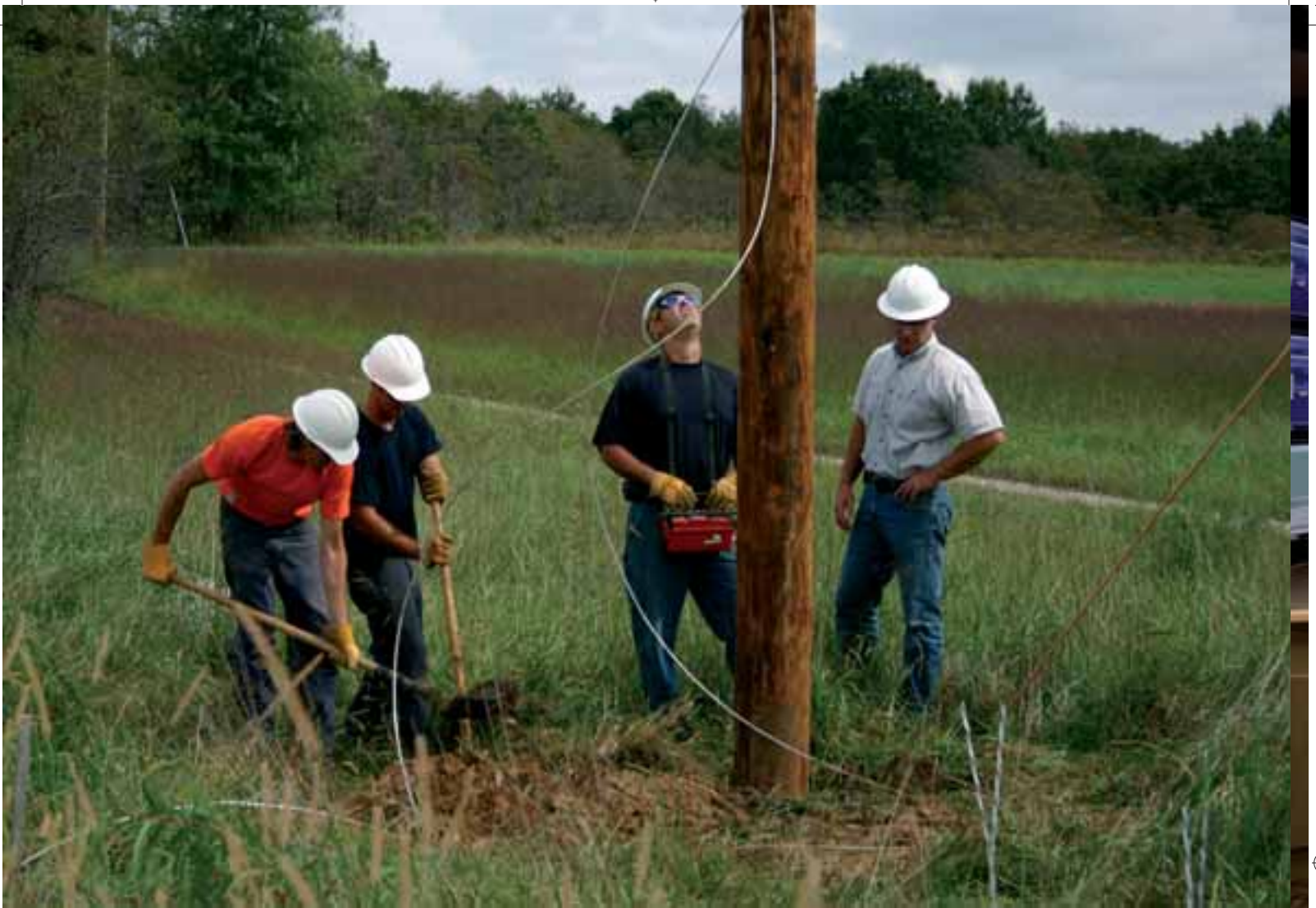
Line Superintendent Randy Long oversees a new service being built.
