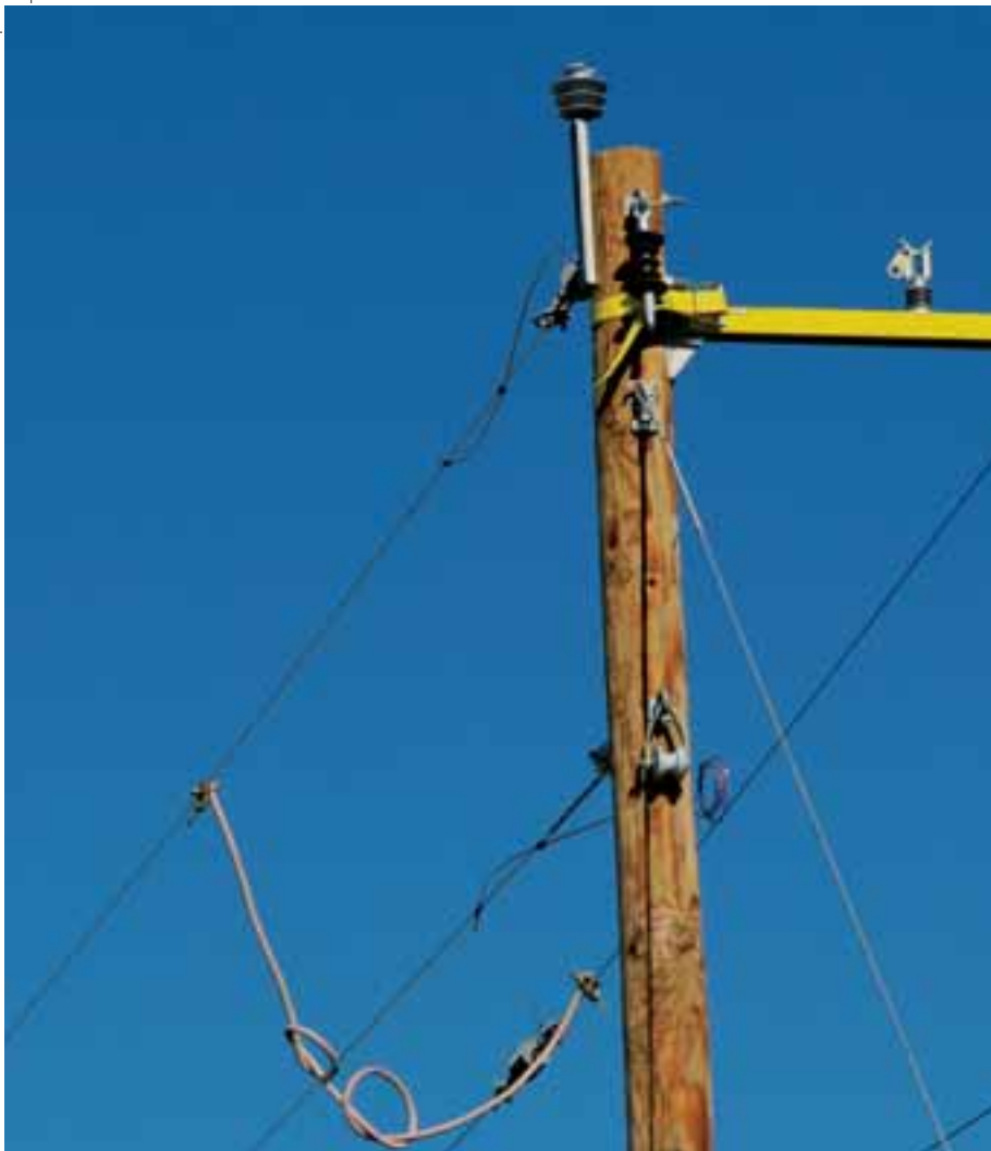
Above, a new single phase line and pole is set.
