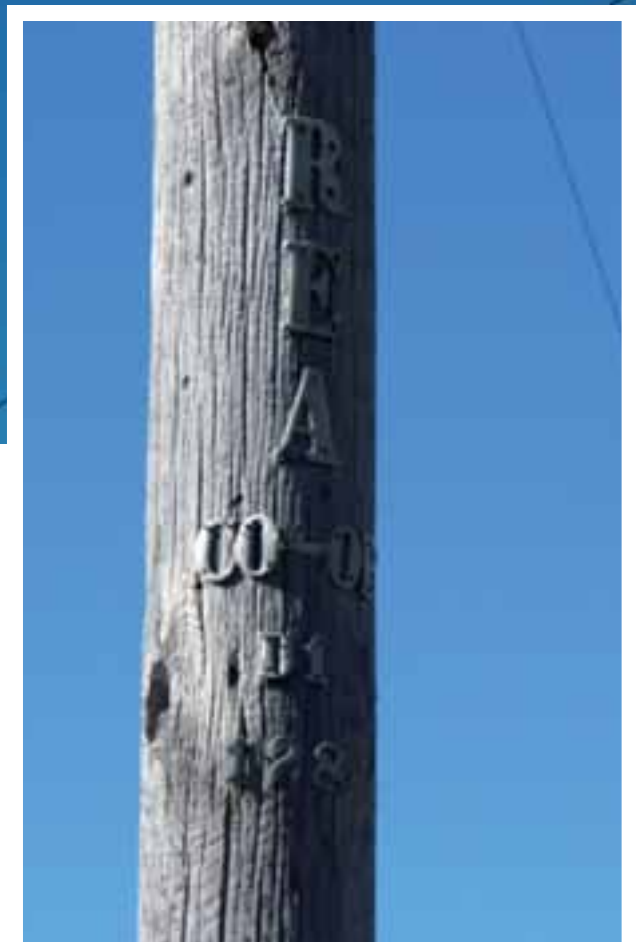
Many of the current poles are over 60 years old.
