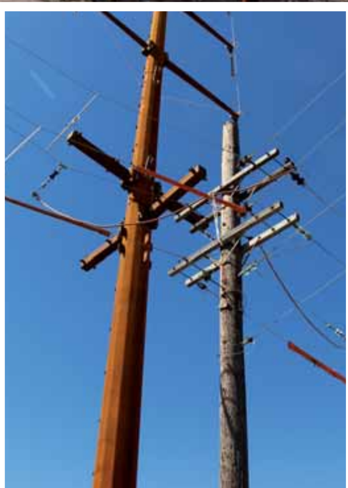
Transmission poles being replaced on the Hillview blacktop near Winchester.
