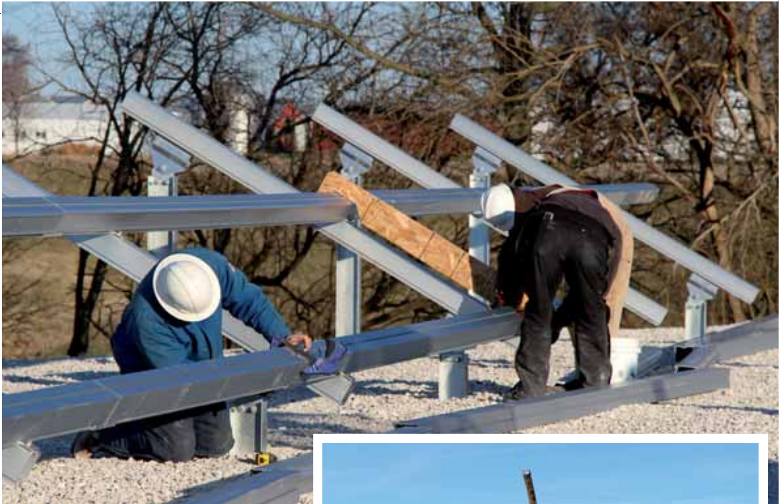
Bigelow Electric installing the mounts for the solar panels.
