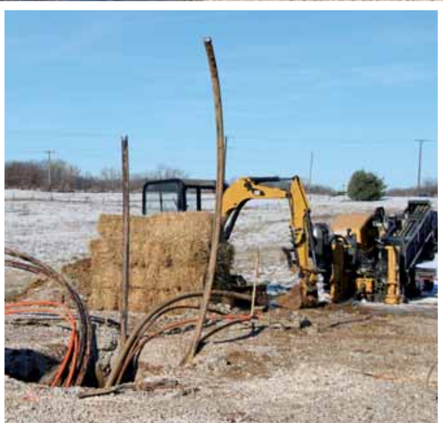
Conduit being trenched for the underground electrical connections.
