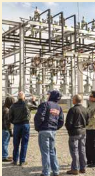
EnerStar board members and employees take cooperative training into the field to see the new Martinsville substation.
