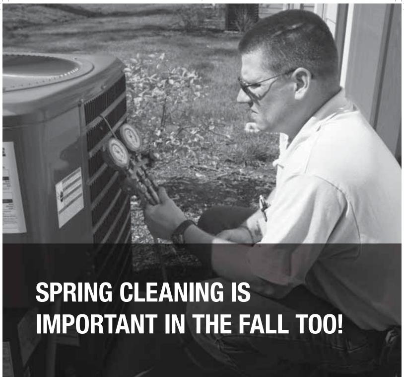
Making sure the coils on your heat pump are clean helps reduce energy consumption and reduces equipment failure. Having a professional technician perform a regular 'check and clean' can ensure your heat pump works at peak efficiency this winter. Make sure the electricity to the unit is turned off before performing any maintenance tasks.
