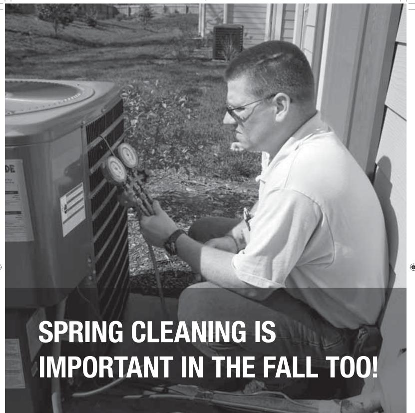
Making sure the coils on your heat pump are clean helps reduce energy consumption and reduces equipment failure. Having a professional technician perform a regular 'check and clean' can ensure your heat pump works at peak efficiency this winter. Make sure the electricity to the unit is turned off before performing any maintenance tasks.
