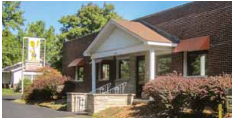
Current Murphysboro office located on Old Highway 13, between Murphysboro and Carbondale.
