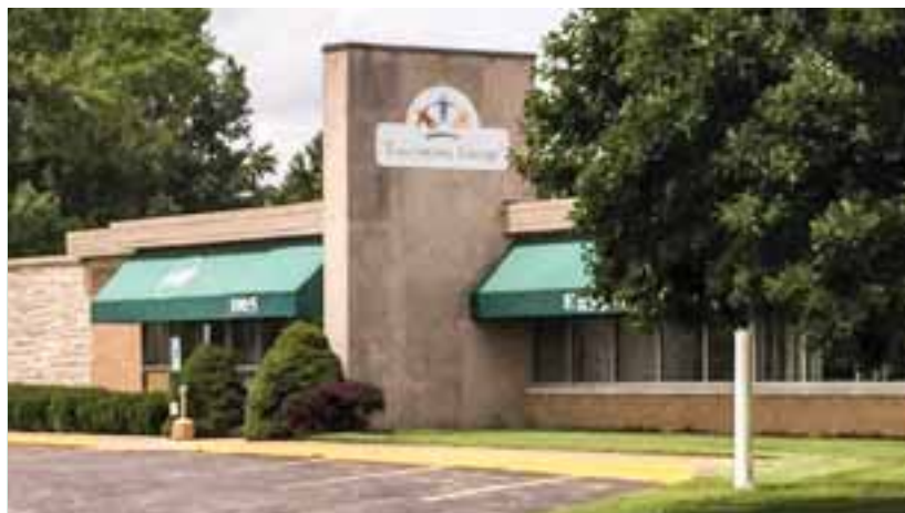
Existing Steeleville facility located on Route 4, on the west side of Steeleville.
