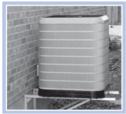
To make sure this doesn't happen to you, occasionally verify that the outdoor unit is running when the system inside is. If not, you may have a unit that has failed and you may need to call a repairman. Before doing that though, double check the thermostat to make sure no one has inadvertently put the system into emergency heat mode. This setting shuts the outside unit off and lets the electric coils supply all of the heat.
