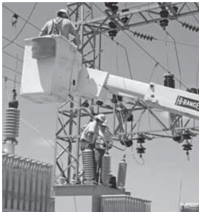
The pictures below and to the right show Clinton County Electric Cooperative Inc. (CCECI) linemen installing a 3750 KVA transformer at our Breese Substation. The addition of this transformer doubles the transformer capacity at the Breese Substation.
