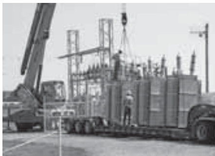
These pictures show CCECI linemen replacing 3 old 833 KVA transformers, with 3 refurbished 1250 KVA transformers at our Bartelso Substation. Increasing the transformer capacity at the Bartelso Substation should allow for growth in the many years to come.
