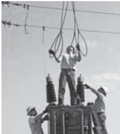
These pictures show CCECI linemen replacing 3 old 833 KVA transformers, with 3 refurbished 1250 KVA transformers at our Bartelso Substation. Increasing the transformer capacity at the Bartelso Substation should allow for growth in the many years to come.
