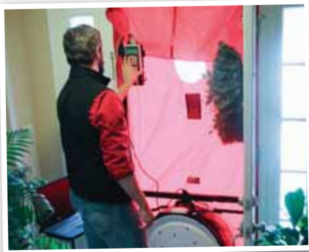
Pictured above: Energy Advisor Justin Stuva checks for potential gas leaks (top) and runs diagnostics on a blower door test (bottom) during a recent home energy audit.
